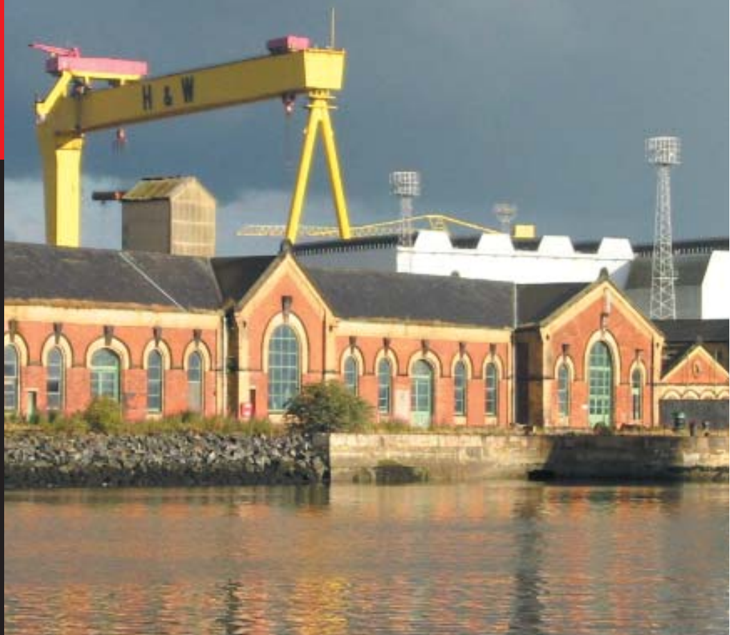
Pictured above: Thompson Dock Pumphouse
