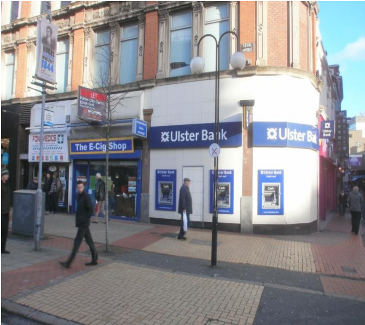
Poor shop frontages, city centre
