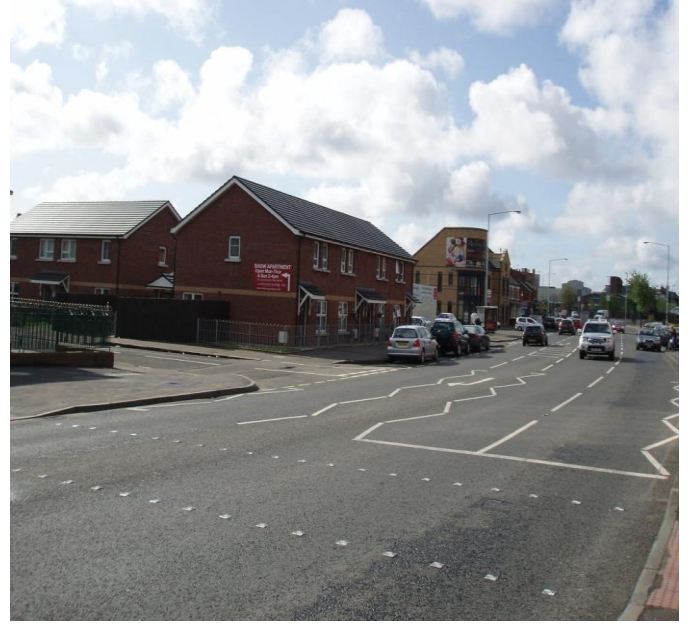
Inappropriate scale / enclosure – Shore Road
